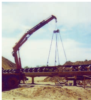
Crane positioning X-ray equipment into position
