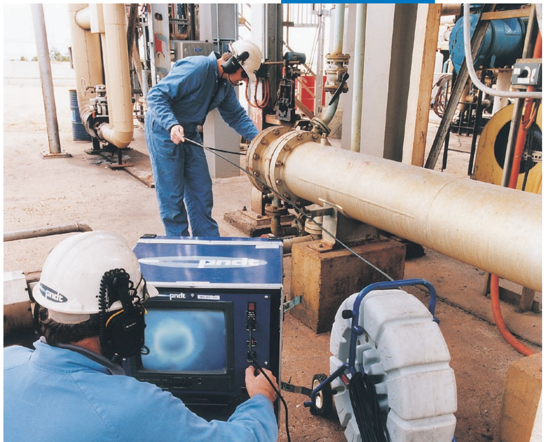
Inspection and VCR recording of plant piping
