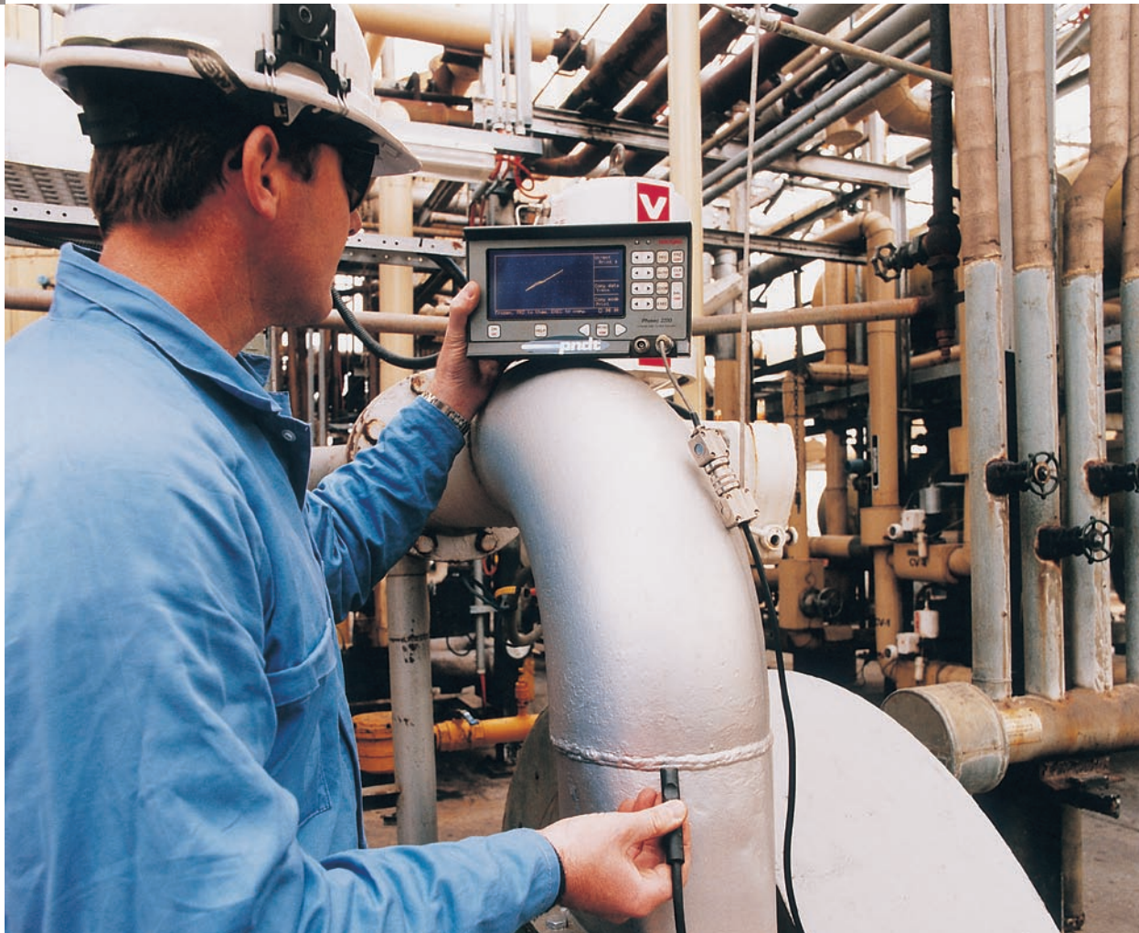
Crack detection of coated weld
